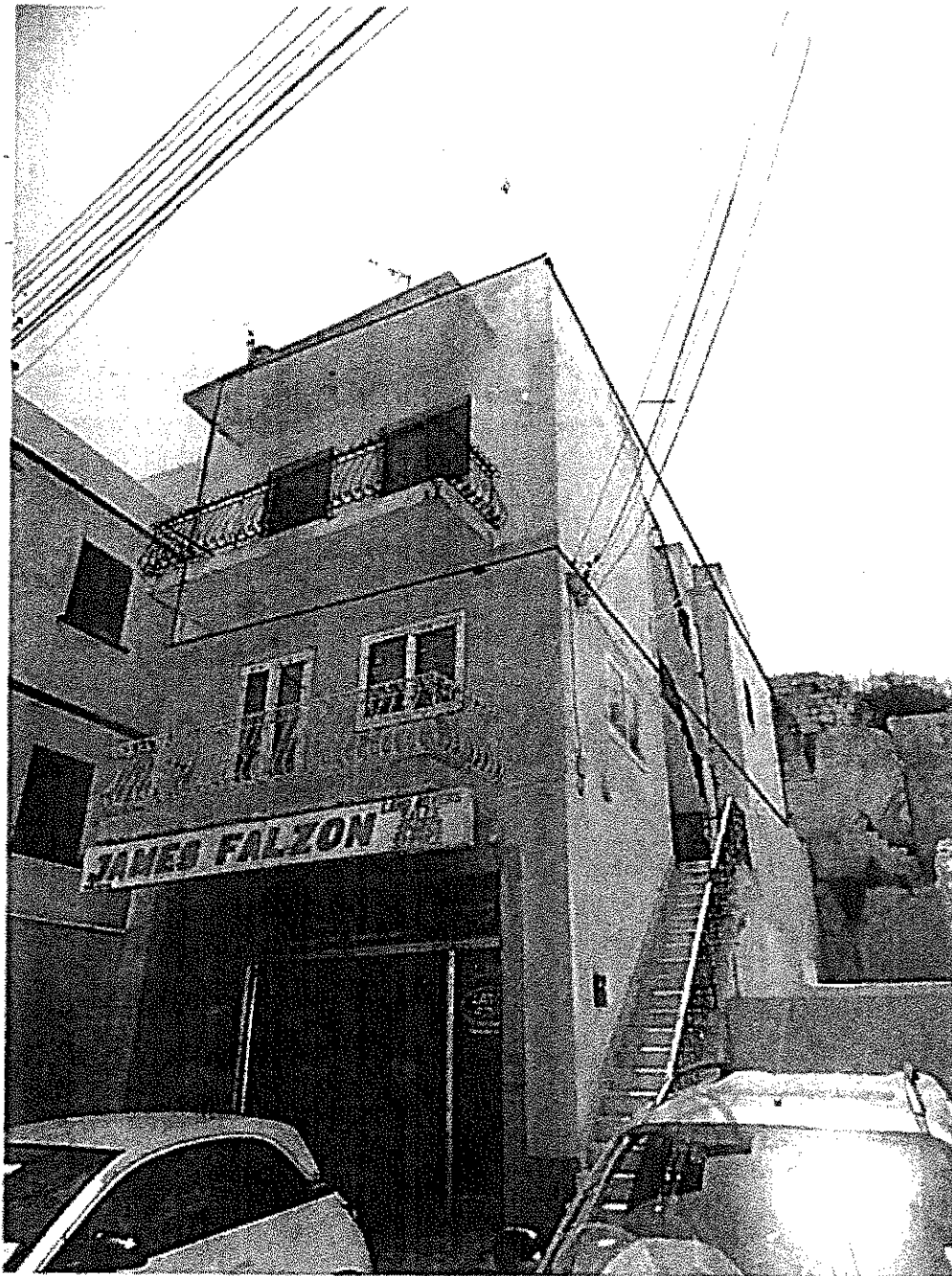
Photo B: Maisnette 2, Edel, GDS Building, Valley Road, Msida
