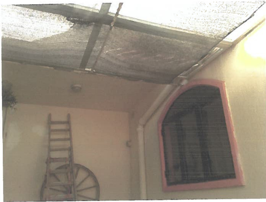
Cod. 391 (that it-terrazzin tal-kamra tas-sodda 2 - mill-ewwel sular)
