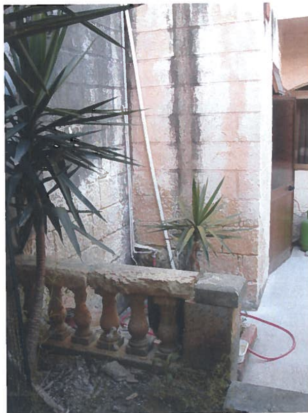
Shower room being used as a store in the backyard.
